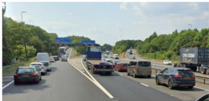
M4 Westbound at J23A Magor showing raised slip road and idling traffic. A typical day of noise and air pollution.
